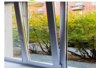
Exterior general metal
